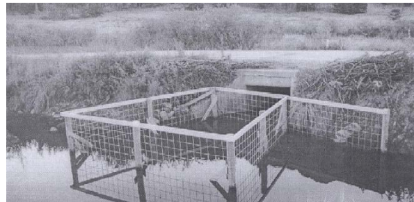
Figure 49: Beaver deceiver (Brown et al. 2001).
