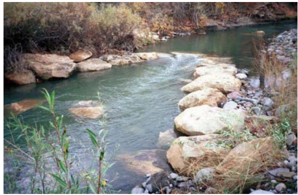
Figure 63: Cross vane on the Rio Blanco, CO (NRCS 2007, Ch11).
