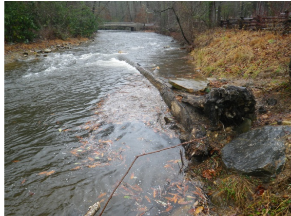
Figure 54: Log J-hook vane providing bank stabilization and pool scour 4 years after construction (Pisgah National Forest, North Carolina; photo credit: Brady Dodd).
