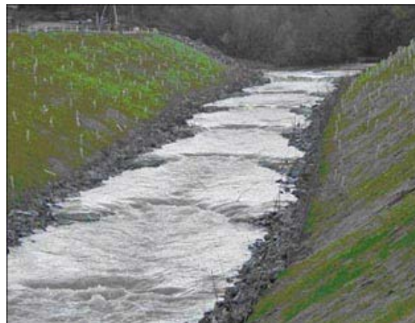
Figure 46: Pool and weir fishway.
