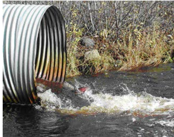
Figure 45: Culvert outlet drop, with Coho.
