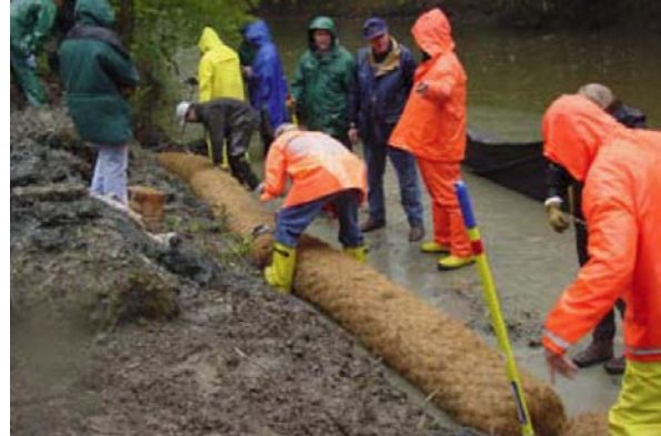
Figure 57: Installation of coir fascines (NRCS 2007, TS14I).
