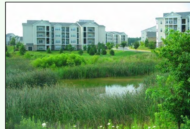
Constructed wetland in Fairfax County Source: Wetland Studies and Solutions, Inc.
