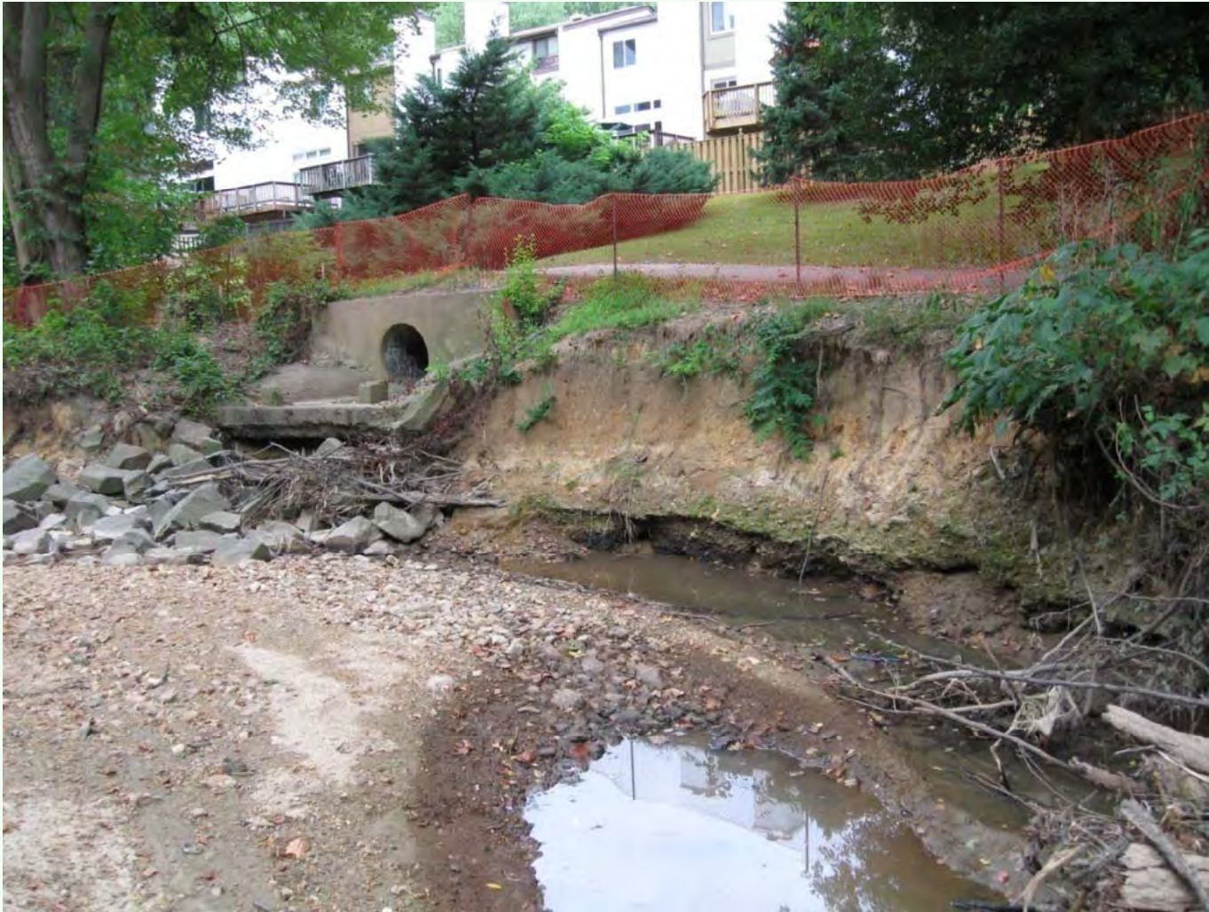
Snakeden Branch in Reston, Virginia, prior to restoration
