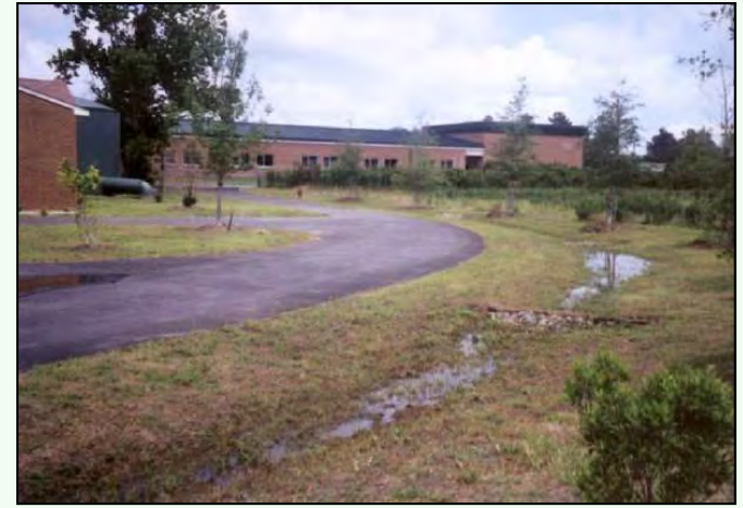
Grass Channel Source: DCR Stormwater Design Spec No. 3
