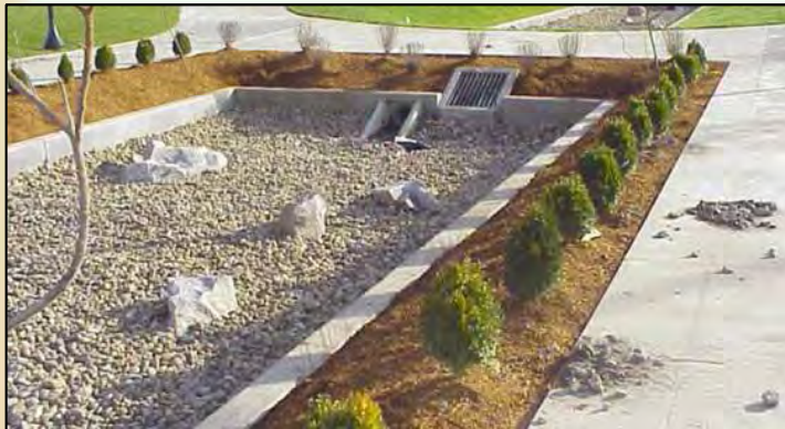
Surface sand filter
