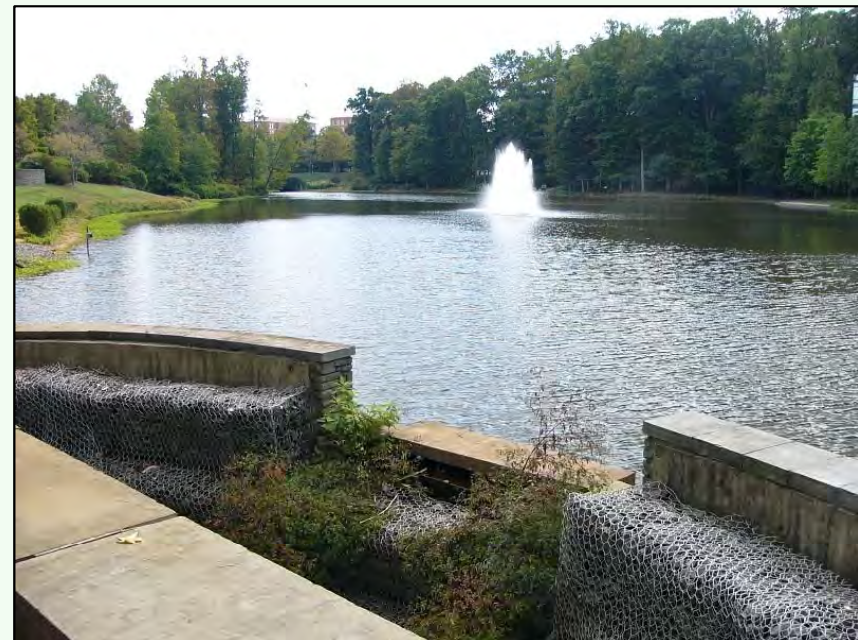
Wet pond in Fairfax County Source: Wetland Studies and Solutions, Inc.
