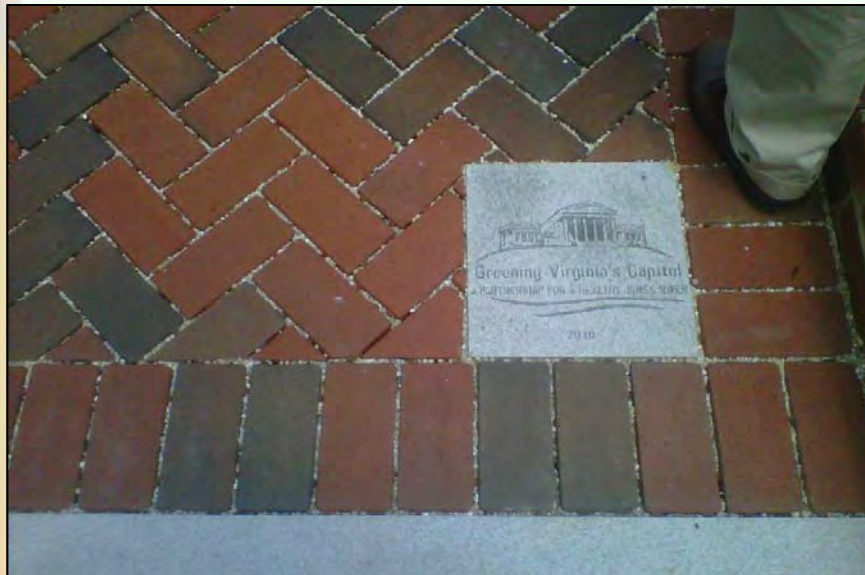
Permeable pavers (brick) at the Virginia Capitol Building Source: Wetland Studies and Solutions, Inc.
