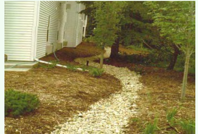
Downspout disconnection and Infiltration trench Source: DCR Stormwater Design Spec No. 8
