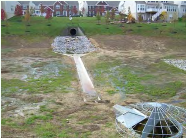
Extended detention pond
