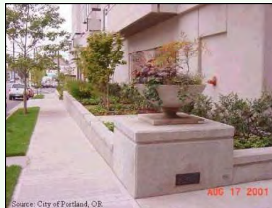
Stormwater planter Source: DCR Stormwater Design Spec No. 9A
