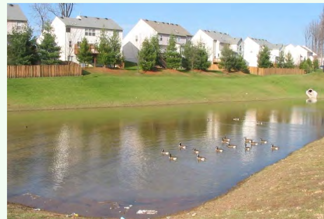
Extended detention pond
