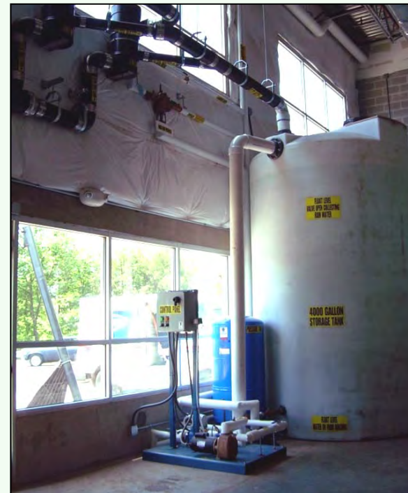
Above-ground rainwater harvesting cistern at WSSI Source: Wetland Studies and Solutions, Inc.
