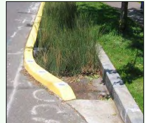
Stormwater curb extension Source: DCR Stormwater Design Spec No. 9A
