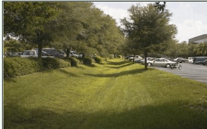
Dry swale Source: DCR Stormwater Design Spec No. 10
