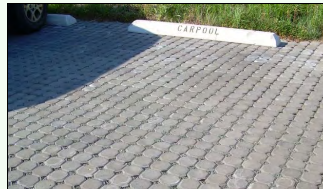
Permeable pavers (concrete) at WSSI Source: Wetland Studies and Solutions, Inc.
