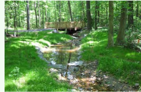
Restored conveyance system
