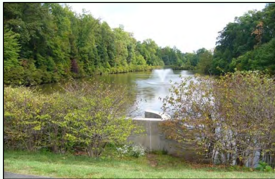
Wet pond in Fairfax County Source: Wetland Studies and Solutions, Inc.
