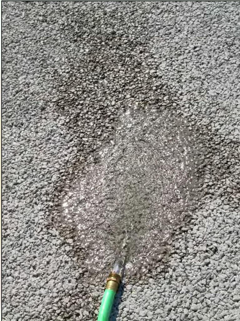
Pervious Concrete at WSSI
