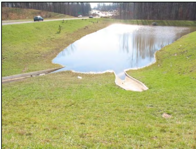
Extended detention in Fairfax County Source: Wetland Studies and Solutions, Inc.
