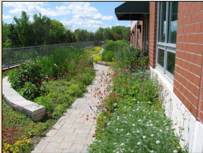
Green roof at WSSI Source: Wetland Studies and Solutions, Inc.
