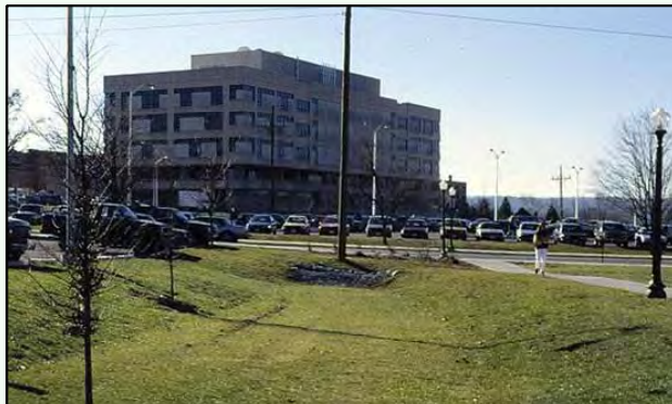
Dry swale Source: DCR Stormwater Design Spec No. 10
