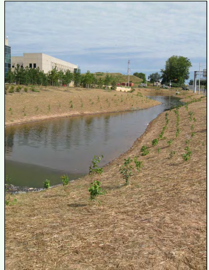
Extended detention in Fairfax County Source: Wetland Studies and Solutions, Inc.
