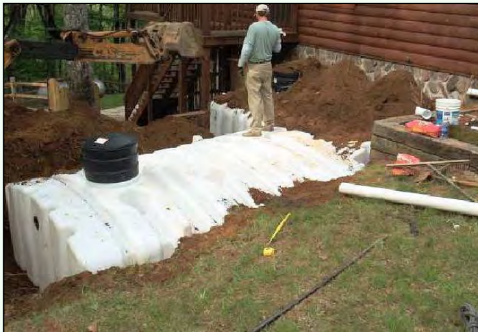
Underground rainwater harvesting cistern Source: DCR Stormwater Design Spec No. 6
