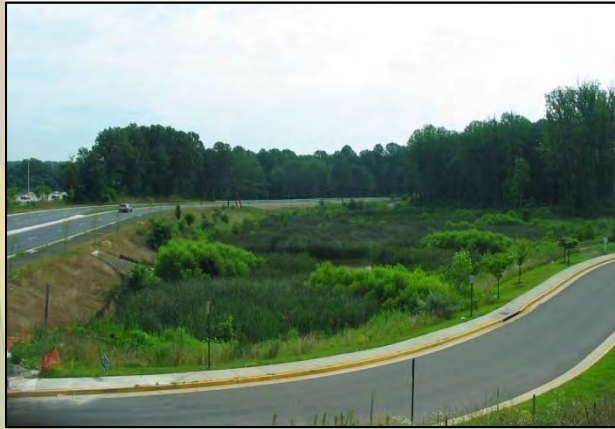
Constructed wetland in Fairfax County Source: Wetland Studies and Solutions, Inc.
