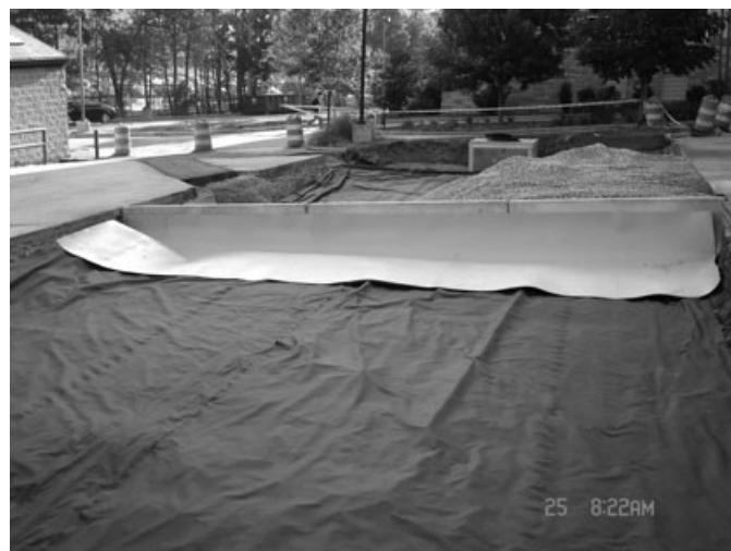
FIGURE 1. Photograph of the Infiltration Beds During Construction. Note the Jersey barrier and geomembrane used to separate the infiltration beds underlying the two pavement types.
